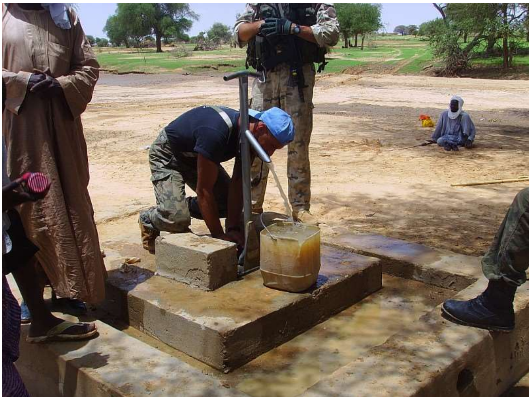
Photo 6. A well built for the civilian population
